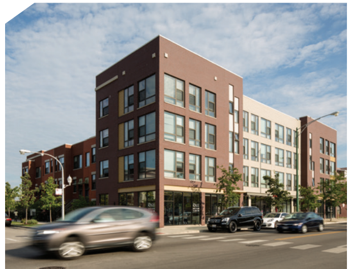
Photo credit: Shane Welch Photography (After: Westhaven Park IIC)
