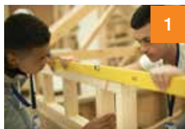
Platform for renewal
